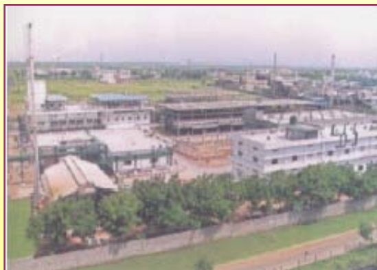
Suryapet Suven Intermediate Mfg. facility
